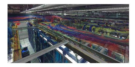
Overloaded cable trays were in danger of structural collapse. Shutting down the data center was not an option. The daunting task included a combination of data capture technologies, workflows and intricate Revit modeling to capture extensive details. PLANiT succeeded in delivering a crucial parametric Revit model to the engineering team for the execution of an
